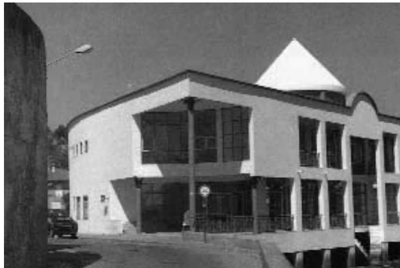
Figure 3.13 Bus Station, Tavira, Portugal
